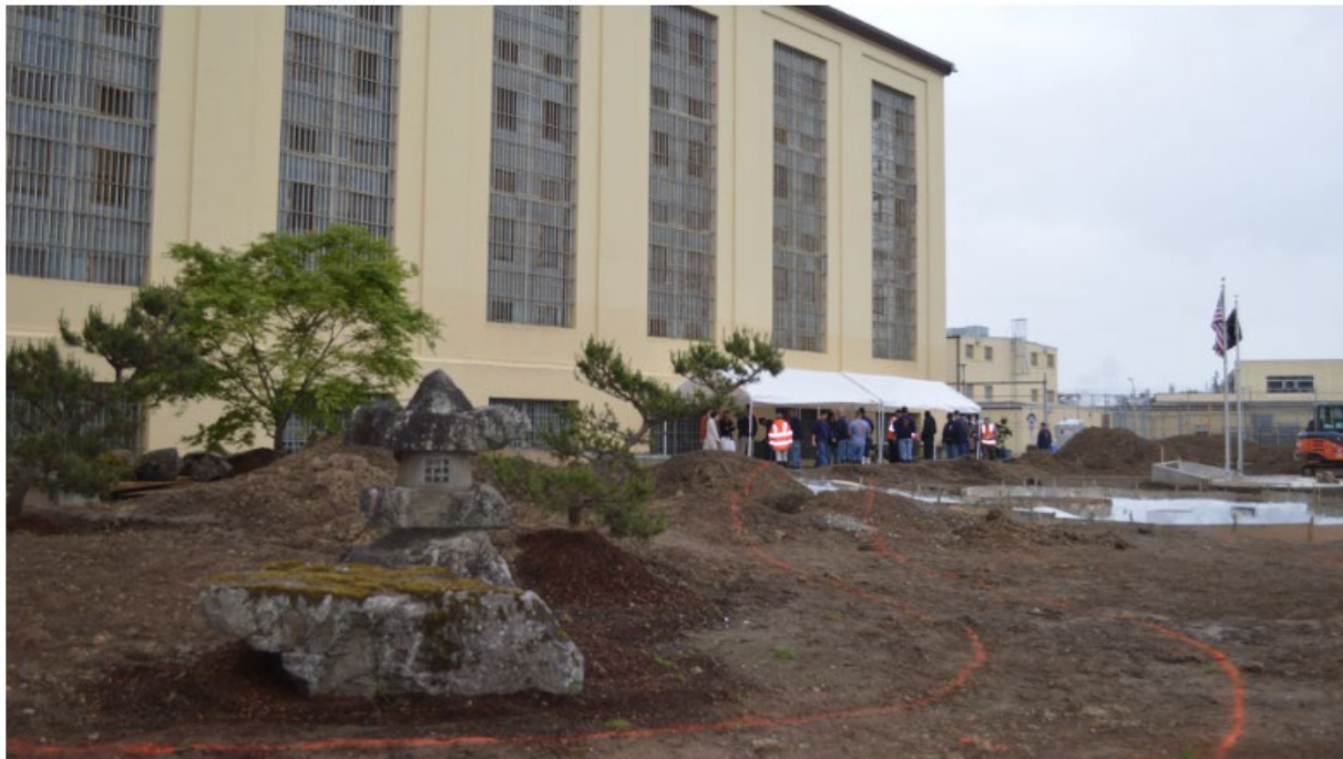
A traditional Japanese garden is under construction in Oregon State Penitentiary.
