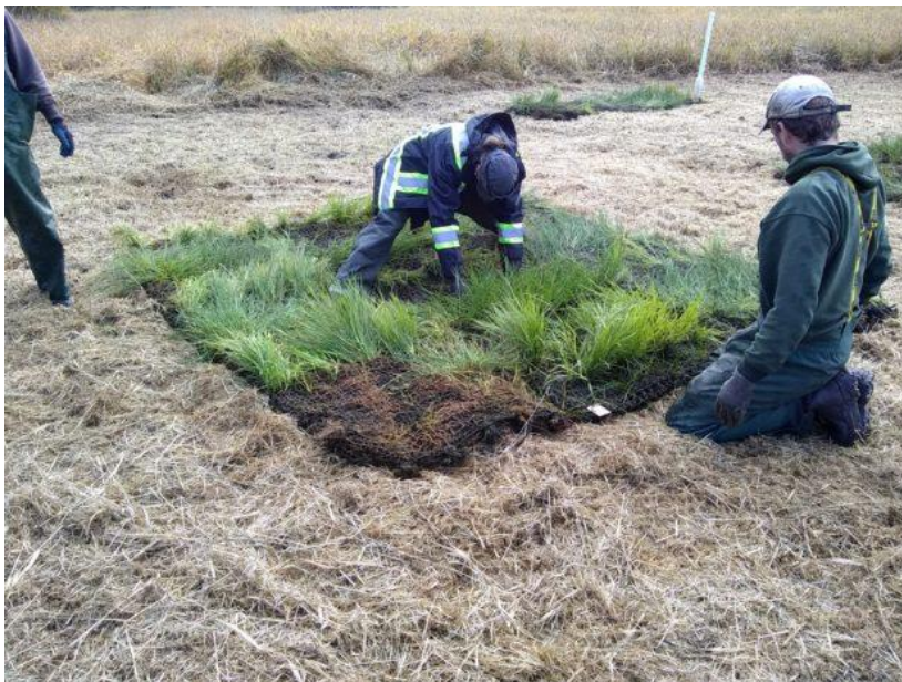
Staff and volunteers from CNLM and JBLM lay three, 1-meter by 3-meter mats side by side and anchor them with biodegradable stakes
