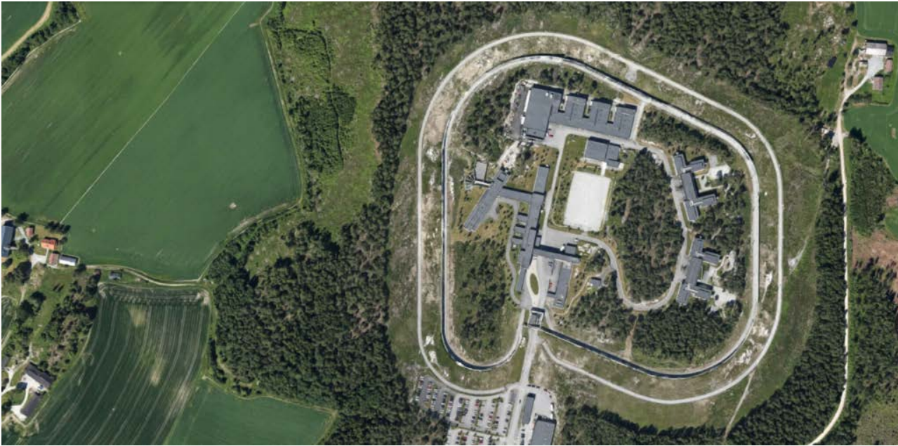
Aerial view of Halden Prison, a campus style prison in Norway with forested grounds.
